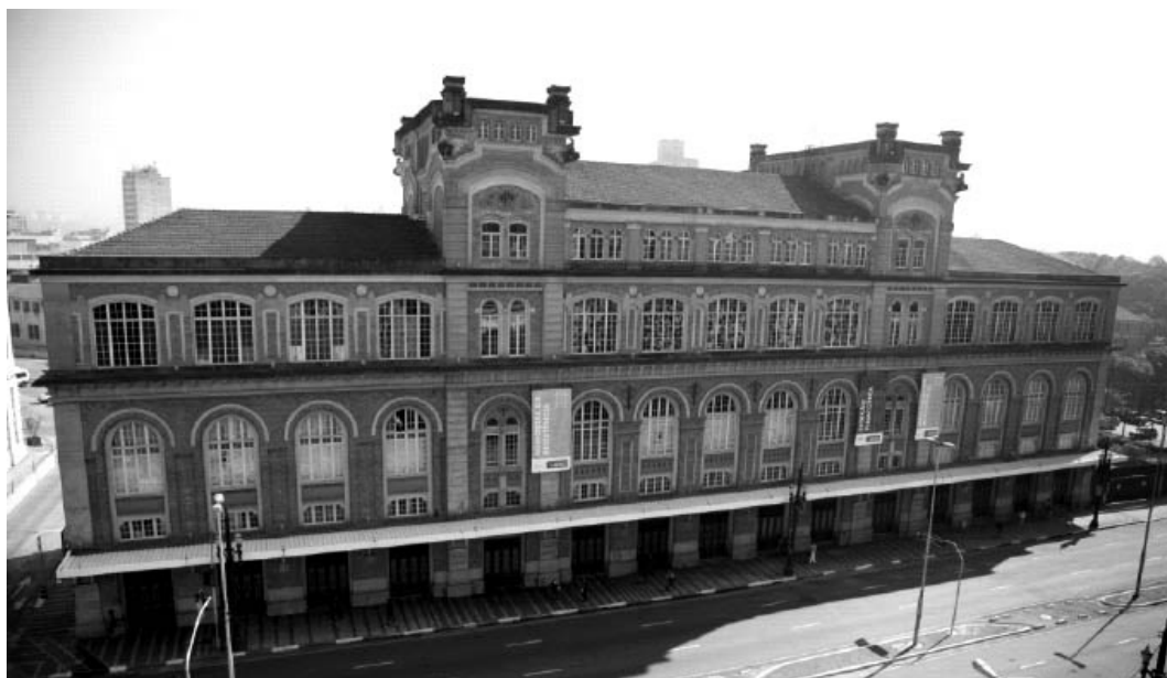
FACADE OF THE OLD STATE DEPARTMENT OF POLITICAL AND SOCIAL ORDER OF SÃO PAULO (DEOPS-SP) BUILDING. PHOTOGRAPH BY PABLO DI GIULIO, MEMORIAL OF RESISTANCE OF SÃO PAULO COLLECTION, 2009.
